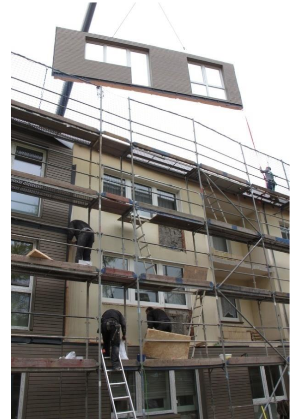
Improving exterior walls renovation
